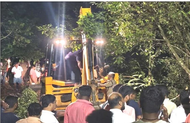
Rescue operation underway after multiple houses collapsed following a mudslide, at Adimali in Idukki district, Kerala---PTI Photo
